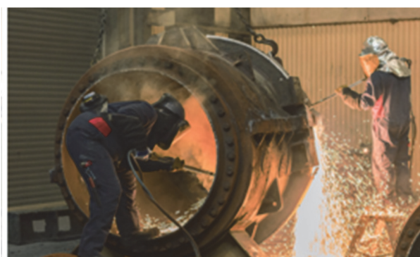
Fig. 5 Thermal segmentation by torch
