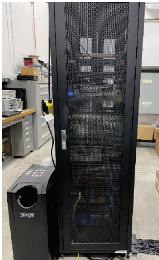
Fig. 2 TRIPP-LITE cooler, shown on the left side, installed into the DAS cabinet
