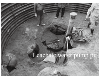
Deformation of leachate bilge pump pit due to the weight of flexible containers
