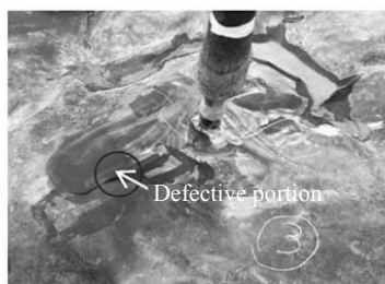
(3) Defective portion around gas vent pipe (after the peeling of cover soil)
