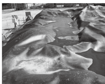
(2) Water pooling due to subsidence
