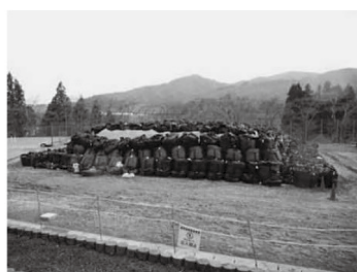
(1) Shifted and collapsed shielding around flexible containers
