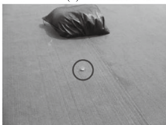
(5) Damage to Protection Mat by Wild Birds (circled)
