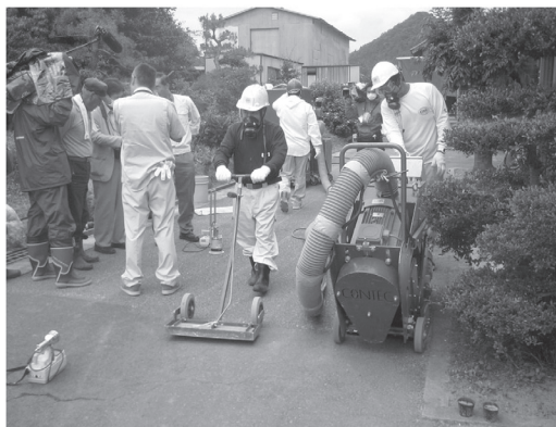
Figure 3 A shot blast for chipping away the surface of asphalt and concrete (photo courtesy of ATOX Co., Ltd.)
