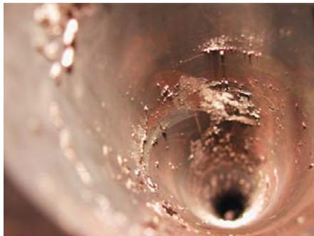
Figure 3. The inside view of the pipe after the operation at low oxygen concentration.
