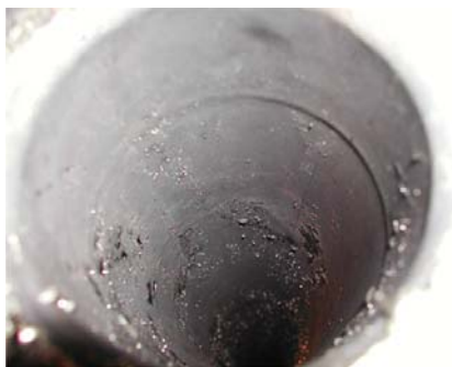
Figure 4. The inside view of the pipe after the operation at middle oxygen concentration.
