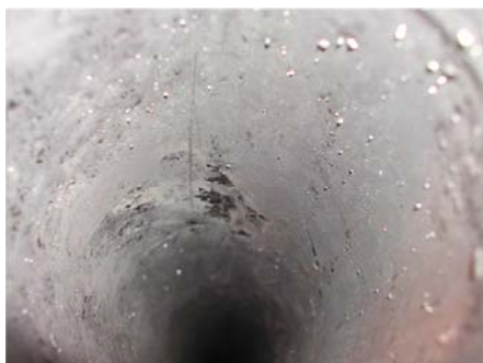
Figure 5. The inside view of the pipe after the operation at high oxygen concentration.
